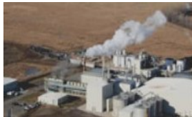
Chippewa Valley Ethanol Coop (CVEC) —Benson CVEC works jointly with the University of MN, Morris studying corn cobs for each of their biomass gasifiers
