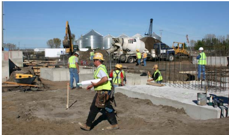
Construction of FibroMinn plant
